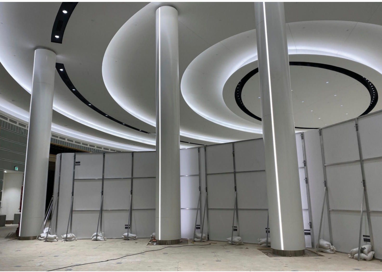
White powder coated Column Covers throughout a large luxury retail mall. Over 200 columns ranging from 10' to 30' in height, some including lighting strips.
