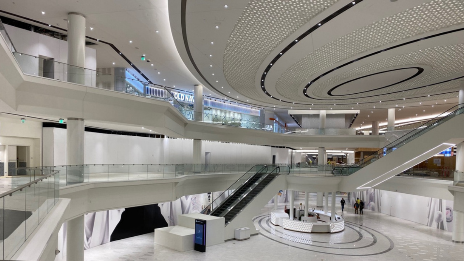
White powder coated Column Covers throughout a large luxury retail mall. Over 200 columns ranging from 10' to 30' in height, some including lighting strips.
